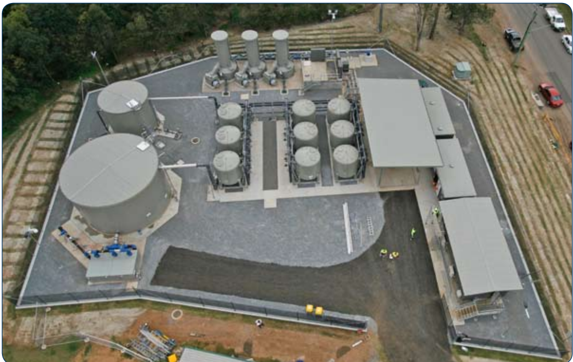
Brisbane Water, Runcorn Water Treatment Plant Copyright 2007 Brisbane Caboolture Aquifuture Alliance Photo courtesy of Brisbane City Council
